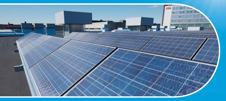
Solar electricity system installed on a solar inverter factory roof in Helsinki, Finland. The main purpose of the system is to provide real life conditions for inverter testing. The design of the system enables connection of different combinations of module strings to one or many inverters, according to the product development needs of the factory. The modules have been installed by using a light-weight, easy to install structure that does not require any penetration through the roof.
