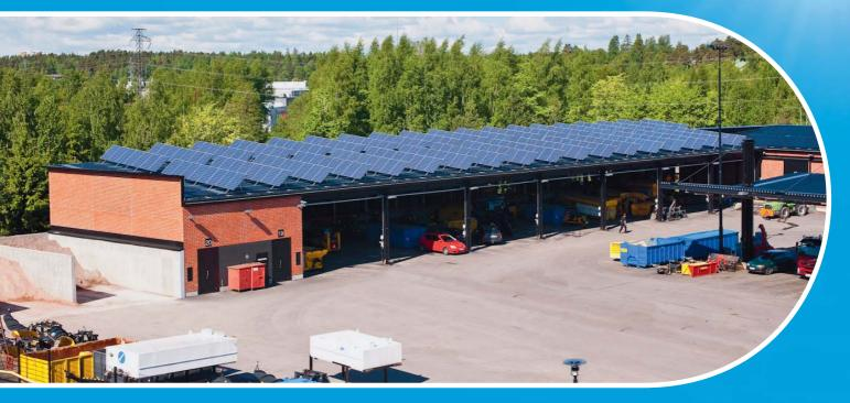
Solar electricity system designed and delivered to the City of Espoo in Finland for charging of electric vehicles. The output of the system will cover the annual need of the 10-15 electric vehicles of the depot. The system is feeding the internal electricity network of the depot to which the vehicles are connected for charging.
