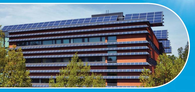
The headquarters of Vaisala were awarded with the golden LEED certification. The required energy efficiency is achieved largely with the building's own electricity generation. One fifth of the electricity need is covered with solar electricity systems installed on the roofs and walls. The arrays are fitted to the architecture of the building with unique mounting structures and with customized solar modules.
