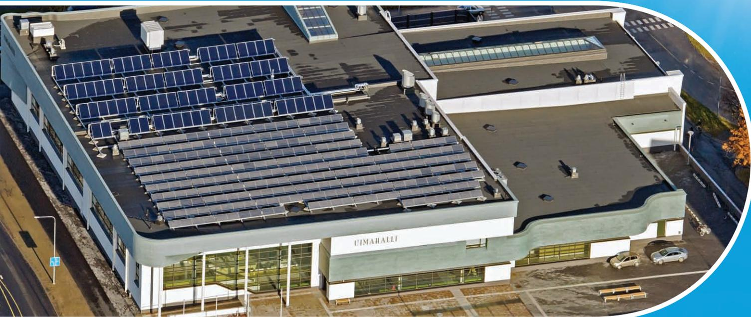
Energy efficiency determined the design work of the new swimming hall at Pori from the very beginning. Several energy-saving technologies have been used. Solar energy is utilized both in heating water and generating electricity. Naps implemented the solar electricity system on the roof with standard solar modules installed on lightweight and easy-to-install aluminium structures. That enabled a quick installation without penetrating the bitumen roof.
